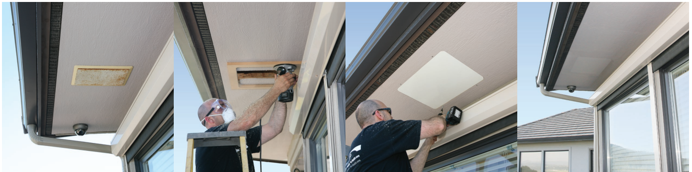
Replace speakers with rusty grilles.
